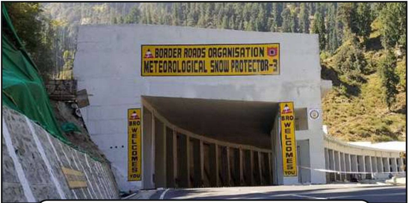
Snow Galleries on Approach Road to South Portal of Atal Tunnel
