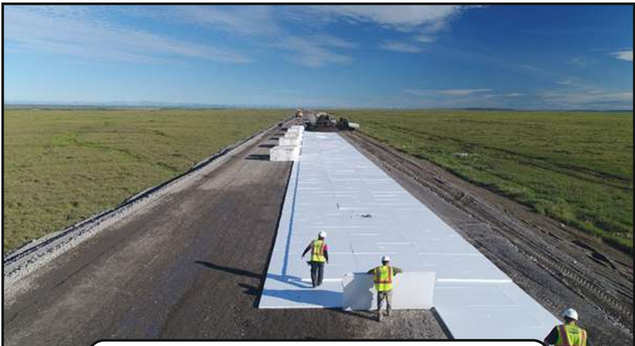
Insulation with Installation of Foam Board
