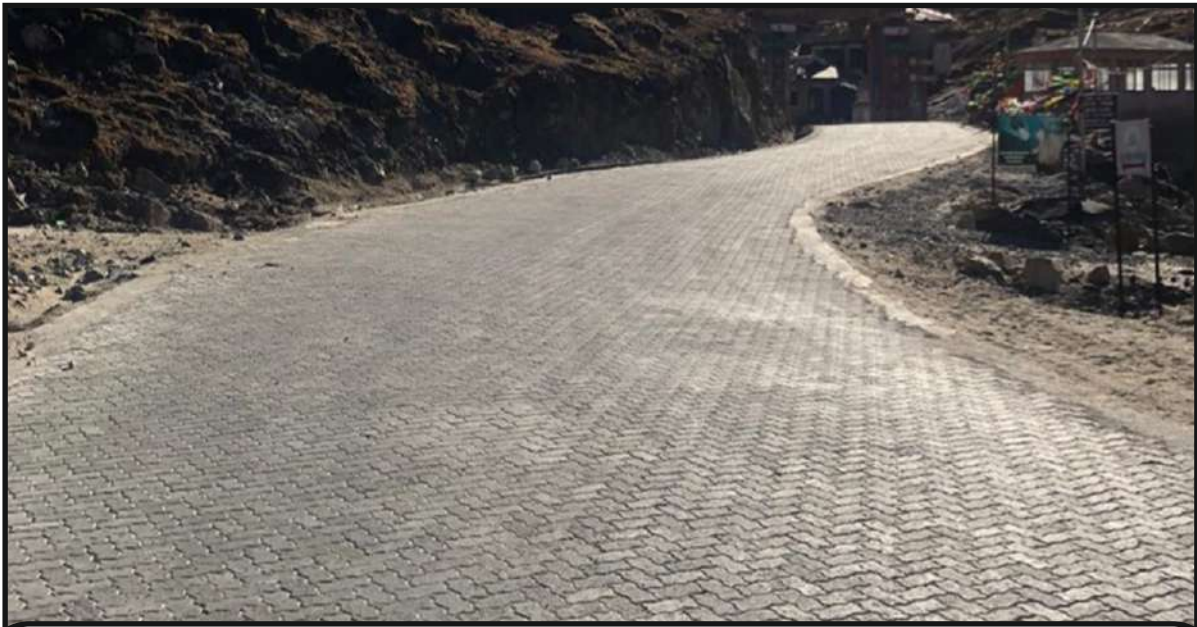
ILCB Pavement on Balipara-Charduar-Tawang Road (Sela Top) in Arunachal Pradesh
