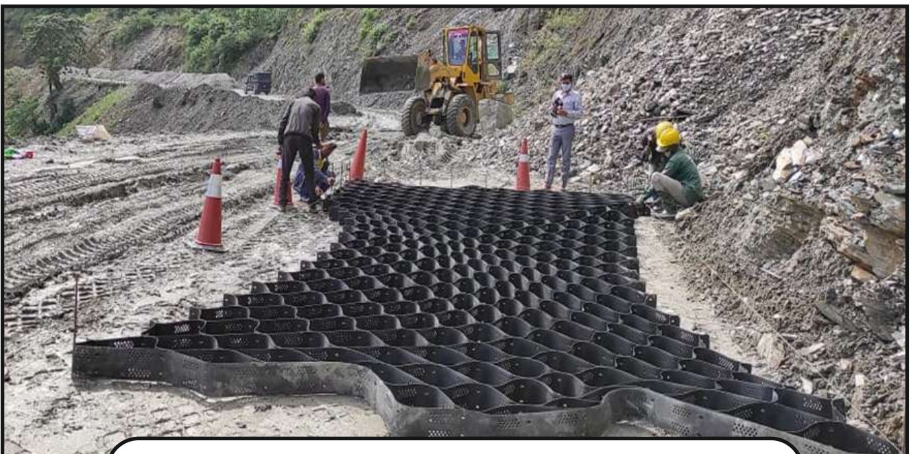
Road Construction with Geo Cell Technology
