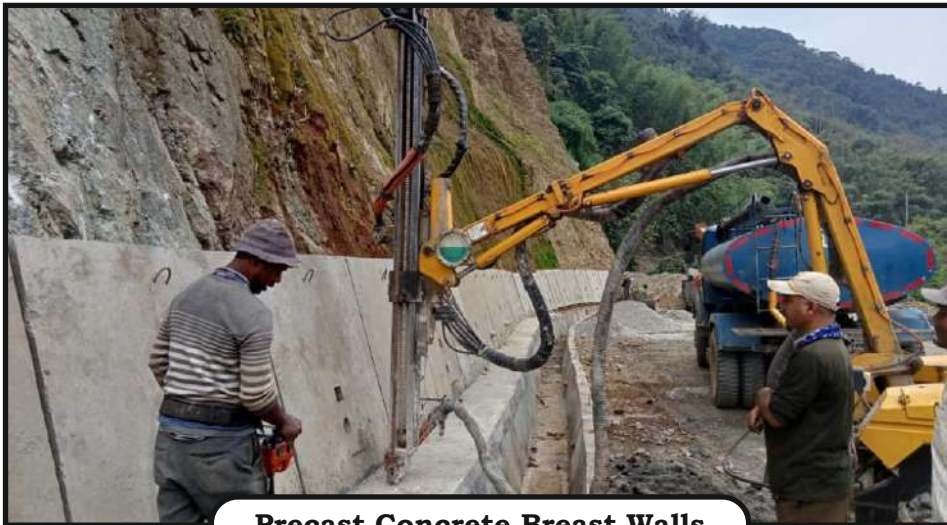
Precast Concrete Breast Walls
